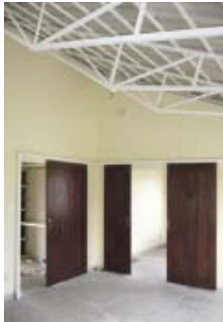
View of the meeting room in the office building in Bukalo.
