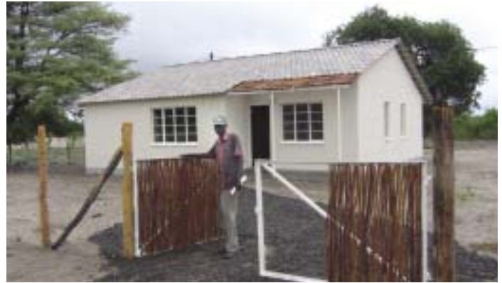
Frontside of the new community forestry structure in Bukalo.
